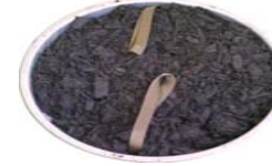
Handles Used For Lifting Screen For Maintenance
